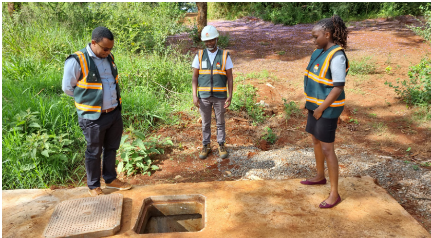
Site visit in Tatu City for the ongoing project
